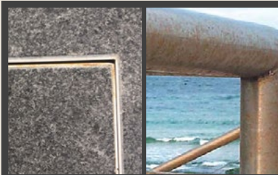
Photo showing 'Tea Staining' on Stainless Steel.
